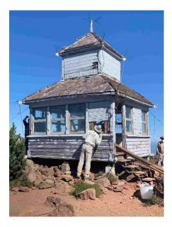
Phase 1 included new roofing, new siding, new shutters, new flooring, repaired supporting structures, and much more. This was completed in October just as the weather was turning and the cupola is now buttoned up and ready for winter.
